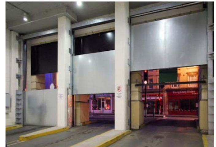
Vehicle and Personnel Door Opening Protection
