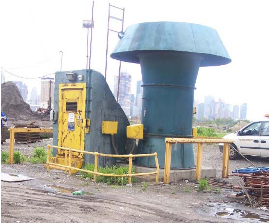
View of 15 th Street Access Shaft
