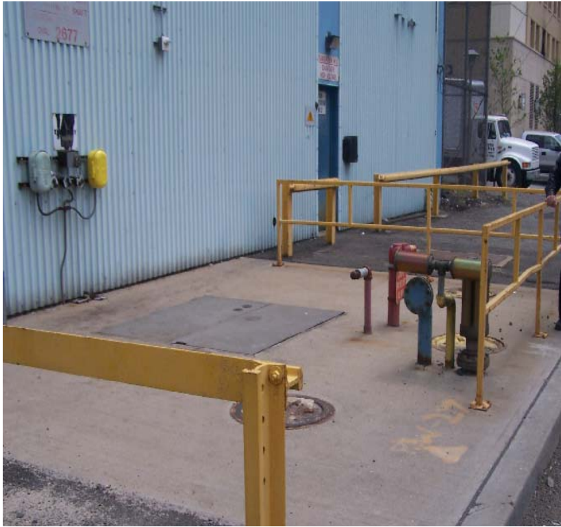
View of Emergency Exit Hatch @ Washington Street Powerhouse
