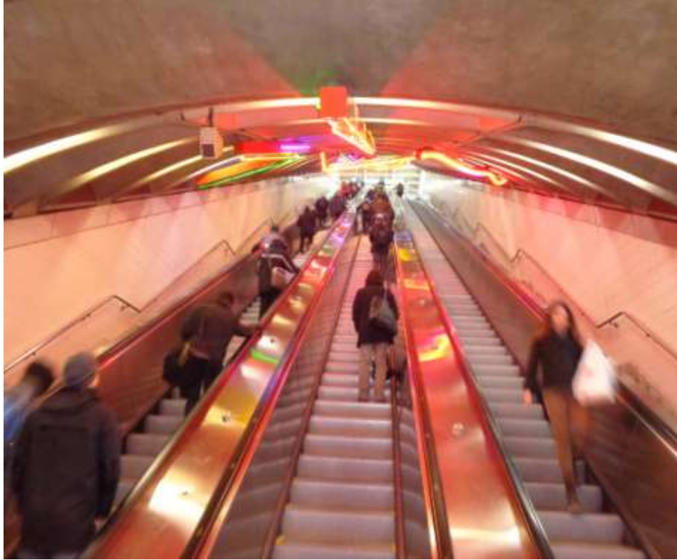
Exchange Place Escalators
